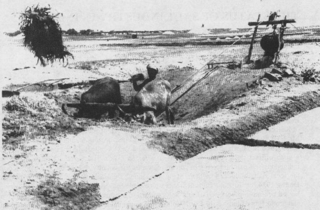
Primitive Method of brine lifiting-using bullocks pair.
